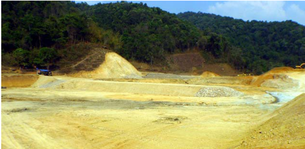
Houay Naking Sediment Management Dam and Sediment Retention Pond under construction – Lao PDR
