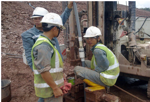
Geotech International performing geotechnical investigation and instrumentation installation at Phu Kham Mine tailings dam using Geotech International Bort Longyear drilling equipment - Lao PDR
