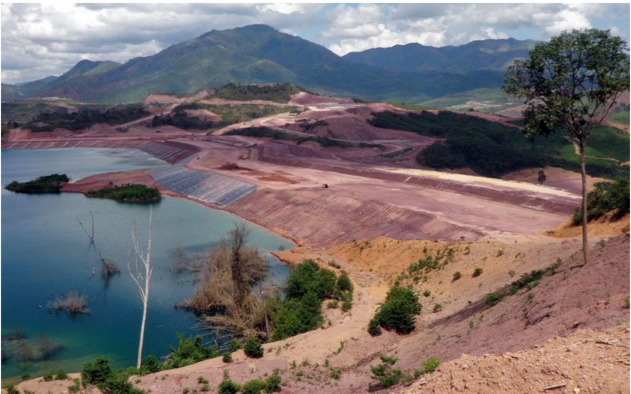
Phu Kham Mine Tailings Dam – Lao PDR
