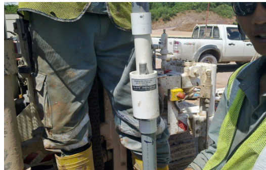
Geotech International performing geotechnical investigation and instrumentation installation at Phu Kham Mine tailings dam using Geotech International Bort Longyear drilling equipment - Lao PDR
