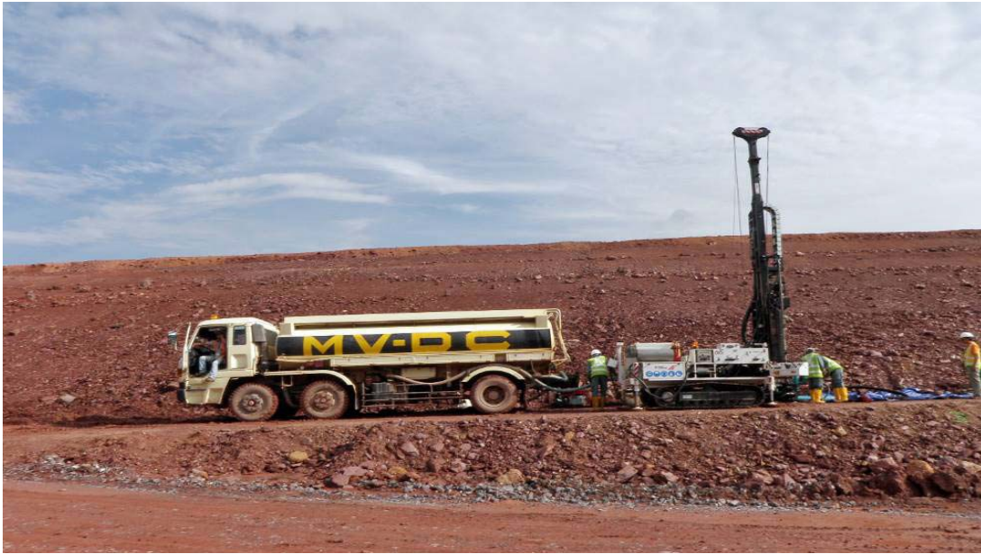
Geotech International performing geotechnical investigation and instrumentation installation at Phu Kham Mine tailings dam using Geotech International Bort Longyear drilling equipment - Lao PDR
