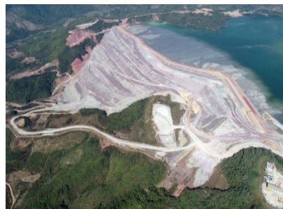
Dam safety instrumentation supply and installation services for one of the largest tailings dams in Asia
