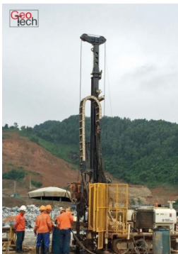
Geotech International Boart Longyear drill performing site investigation for hydropower dam in the Lao PDR
