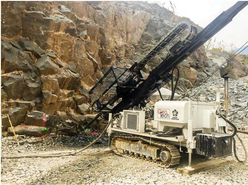
Boart Longyear drilling equipment used to perform the drilling work at grout hole of the BHX TSF Spillway – Lao PDR
