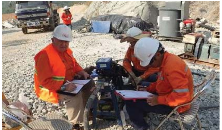
Grout injection in progress performed using DAT instrument readout at the BHX TSF Spillway - Lao PDR
