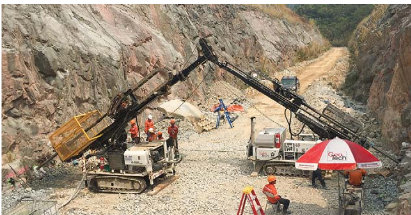
Drilling and Grouting Operation at BHX TSF Spillway – Lao PDR
