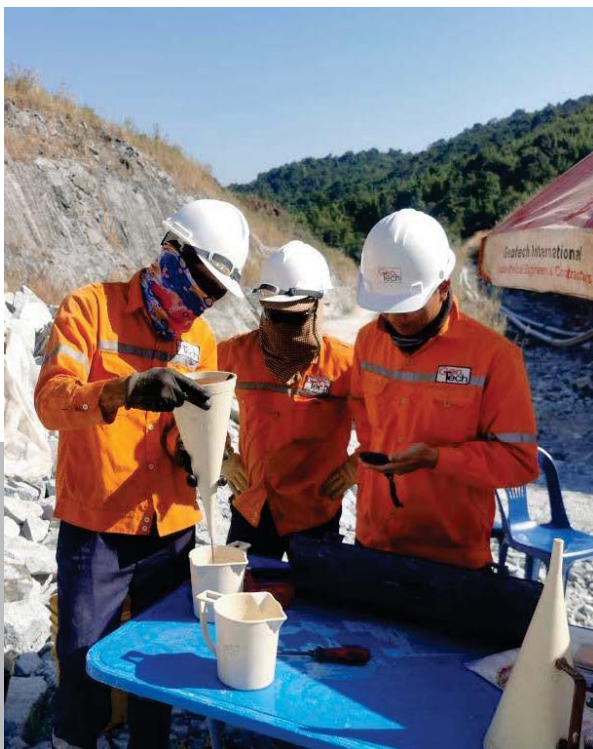
Grout trial mix performed at grouting site
