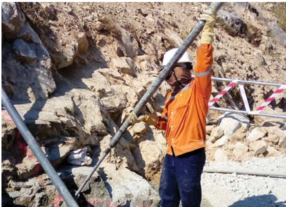
Installation of packer/grout equipment at grout hole on the right abutment of the BHX TSF Spillway
