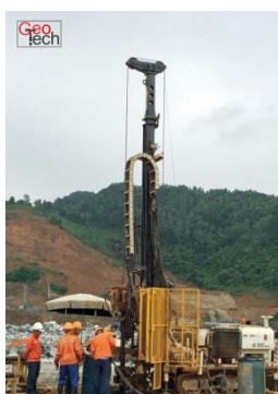
Geotech International Boart Longyear drill performing site investigation for hydropower dam In Lao PDR
