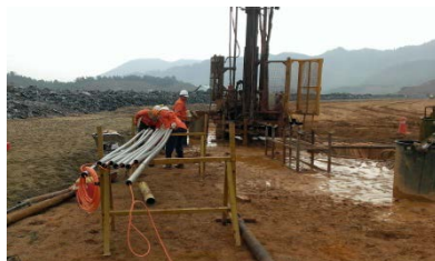
Dam safety instrumentation piezometer, inclinometer and settlement instrumentation for hydropower project in Vietnam
