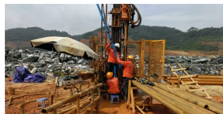
Dam safety instrumentation piezometer, inclinometer and settlement instrumentation for hydropower project in Vietnam
